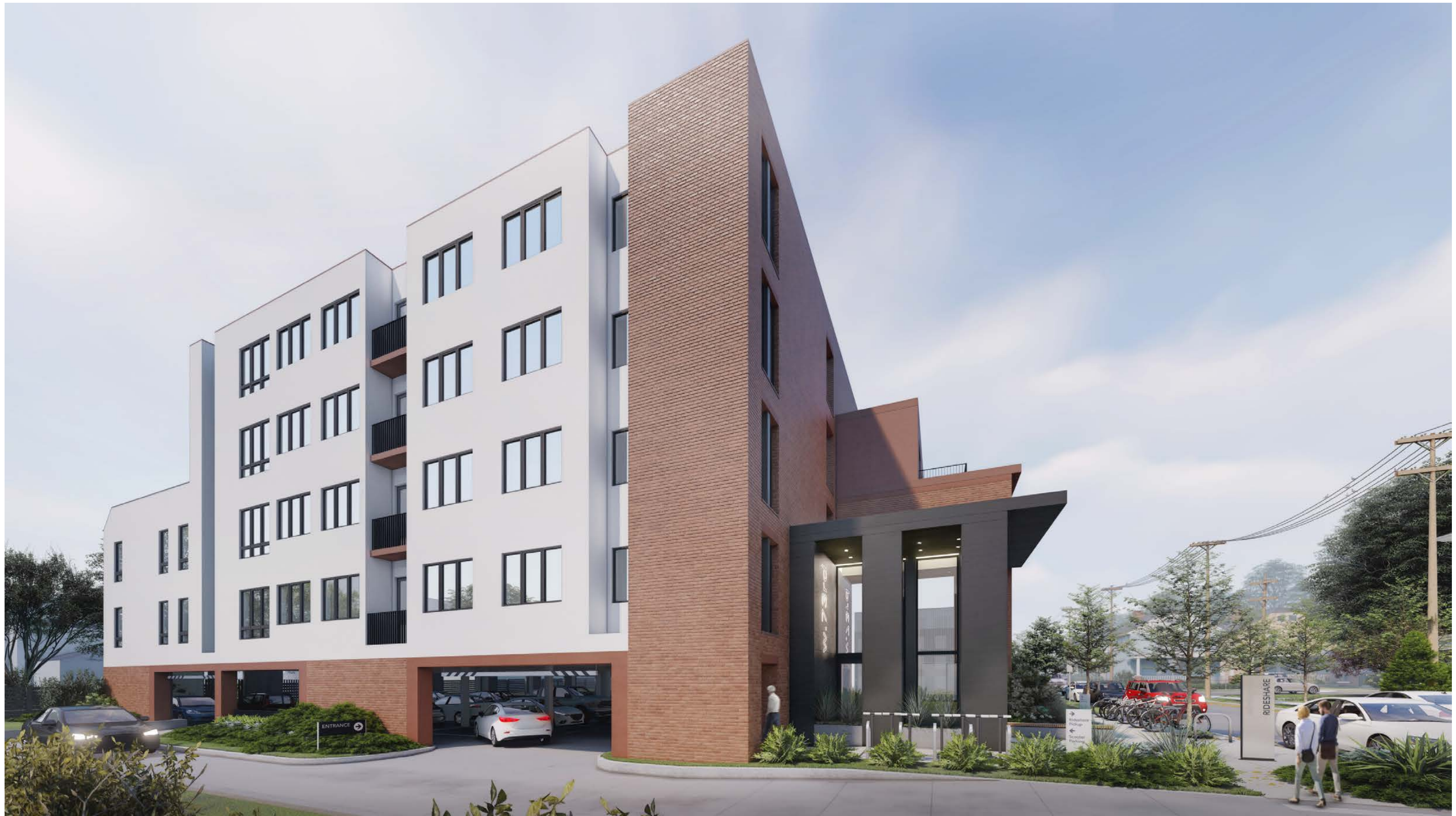
View 13 North Building Side View Showing Parking Garage Entrance
