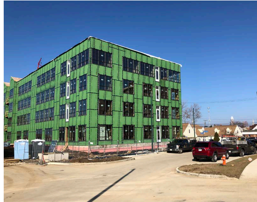
New Construction to the North
