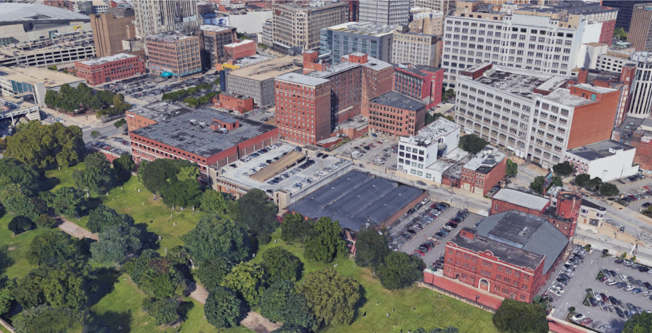
Existing Massing- From Erie Court
