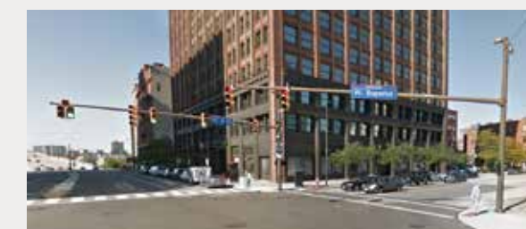
COMBINATION TRAFFIC/STREET LIGHT
