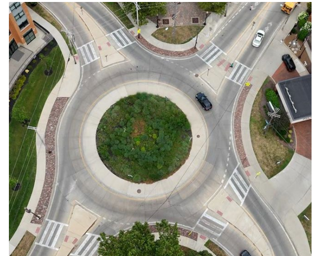
Roundabout example on Franklin Ave. that will be like installation at Ansel Rd.
