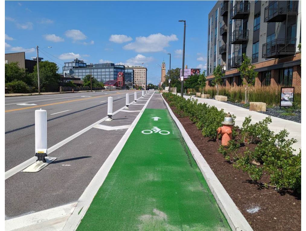
A separated bike lane in Cleveland on Lorain Avenue
