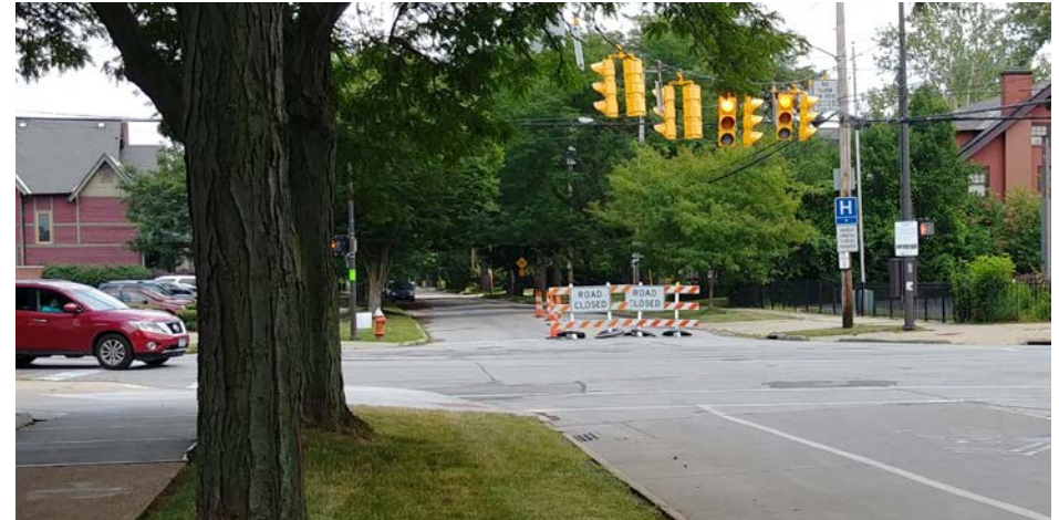
Image 22: Temporary Traffic Diverter at W. 65th St.
