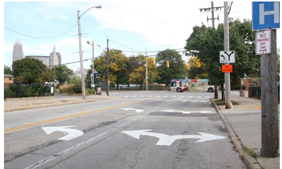
Image 4: Franklin Blvd. at W. 25th St., looking east
