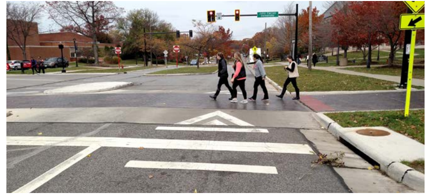
Image 12: Raised Crosswalk, University Heights
