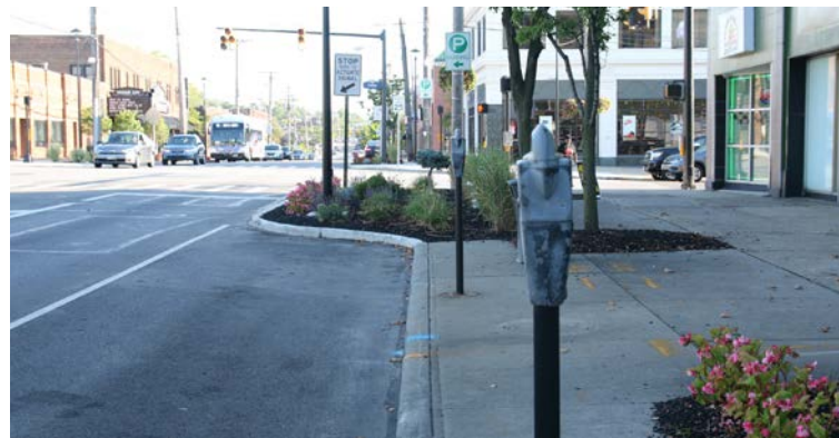
Image 13: Curb extension, Cleveland Heights
