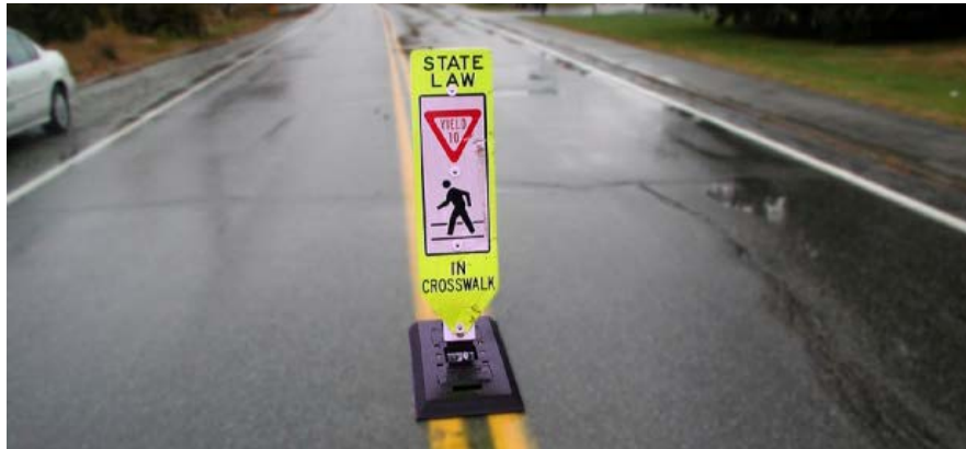
Image 16: In-Street Pedestrian Crossing Sign
