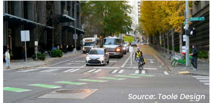
FIGURE 44 Green Paint through intersection.
