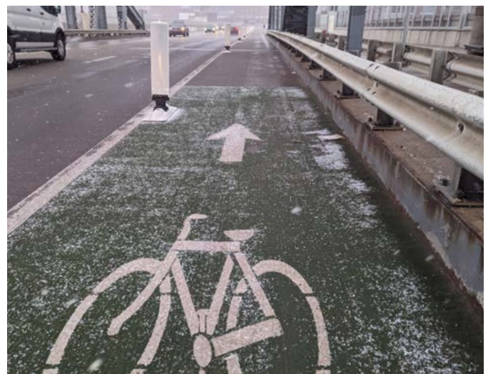
FIGURE 56 Bikeway Seasonal Maintenance.
