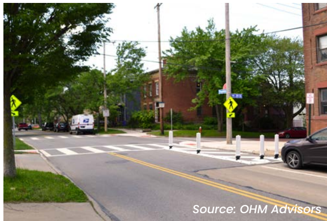
FIGURE 39 Crosswalks on Franklin Boulevard have striped daylighting hardened with plastic delineators.
