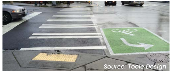
FIGURE 45 Two stage left turn box, similar to the two stage left turn boxes at either end of the Detroit-Superior Bridge.
