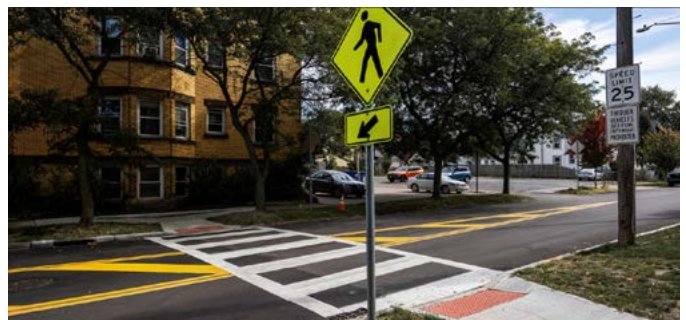
FIGURE 57 ADA-Compliant Sidewalk and Curb Ramp.
