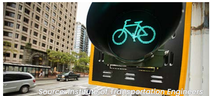
FIGURE 41 Bike Signal, similar to the bike signal at the intersection of the Detroit Superior Bridge and Huron Road for people on bikes going east.
