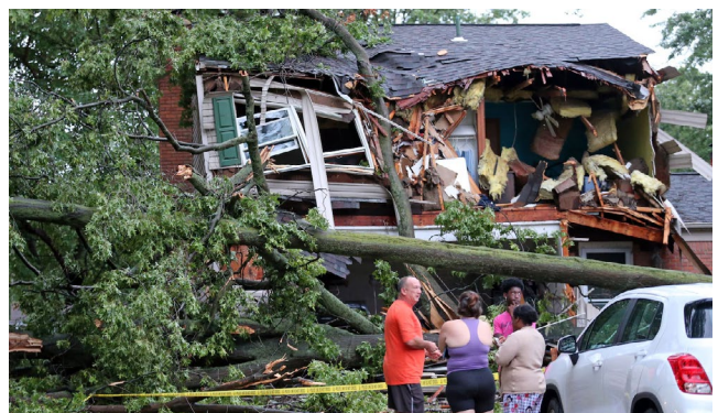
Damage from the August 6, 2024 tornadoes. Courtesy of David Petkiewicz, Cleveland.com.
