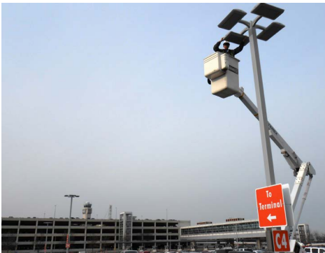
Traditional fixtures being replaced with LEDs at Cleveland Hopkins International Airport.
