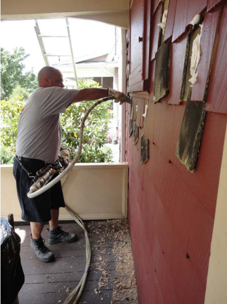
Insulating a Cleveland home as part of the Energy $aver program.
