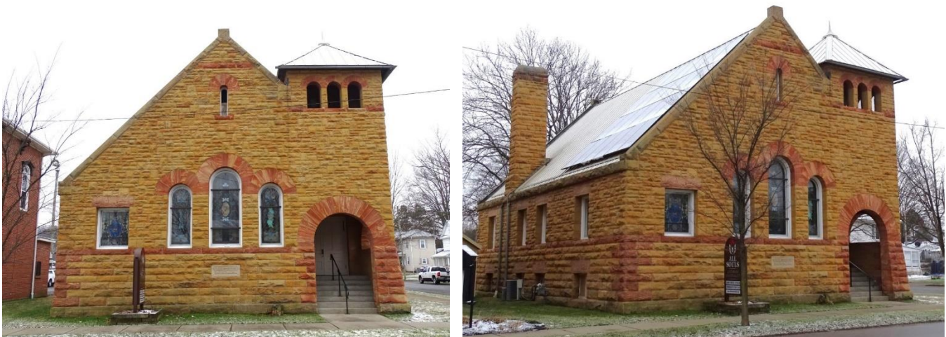
Appropriately placed solar panels should fit with the existing roof and fade into the background.
