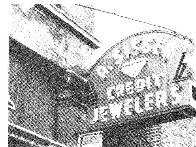
Existing projecting neon sign (to be restored)
