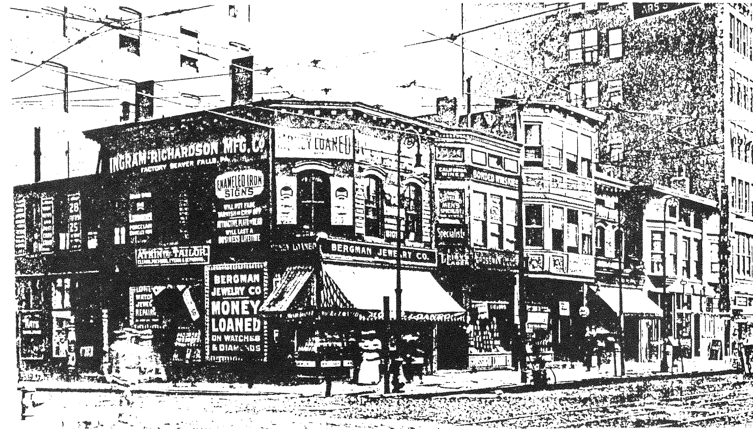
The northeast corner of Prospect & East 4th prior to the construction of the Sincere Building.
