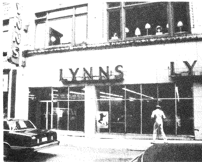
Existing ferro steel panels
