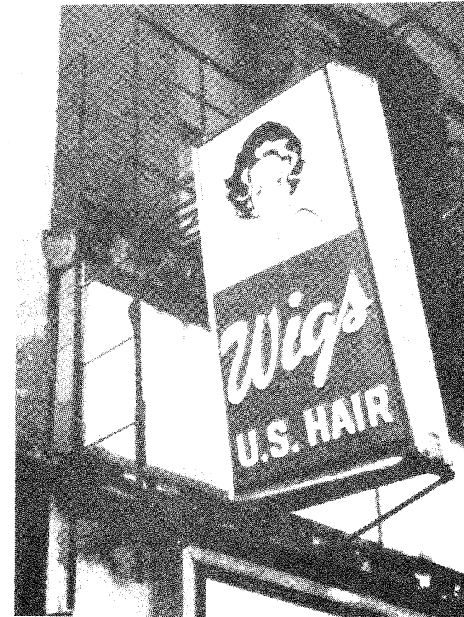
Existing fire escapes should be preserved (Windsor Block)
