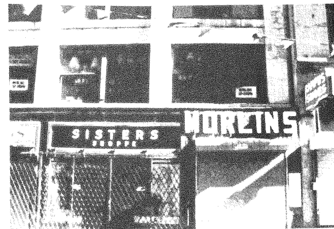
horizontal-sliding steel grilles.
