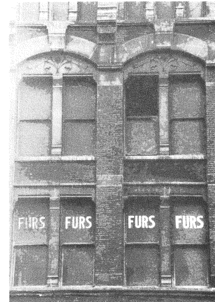
Existing wood windows with signage (to be preserved)
