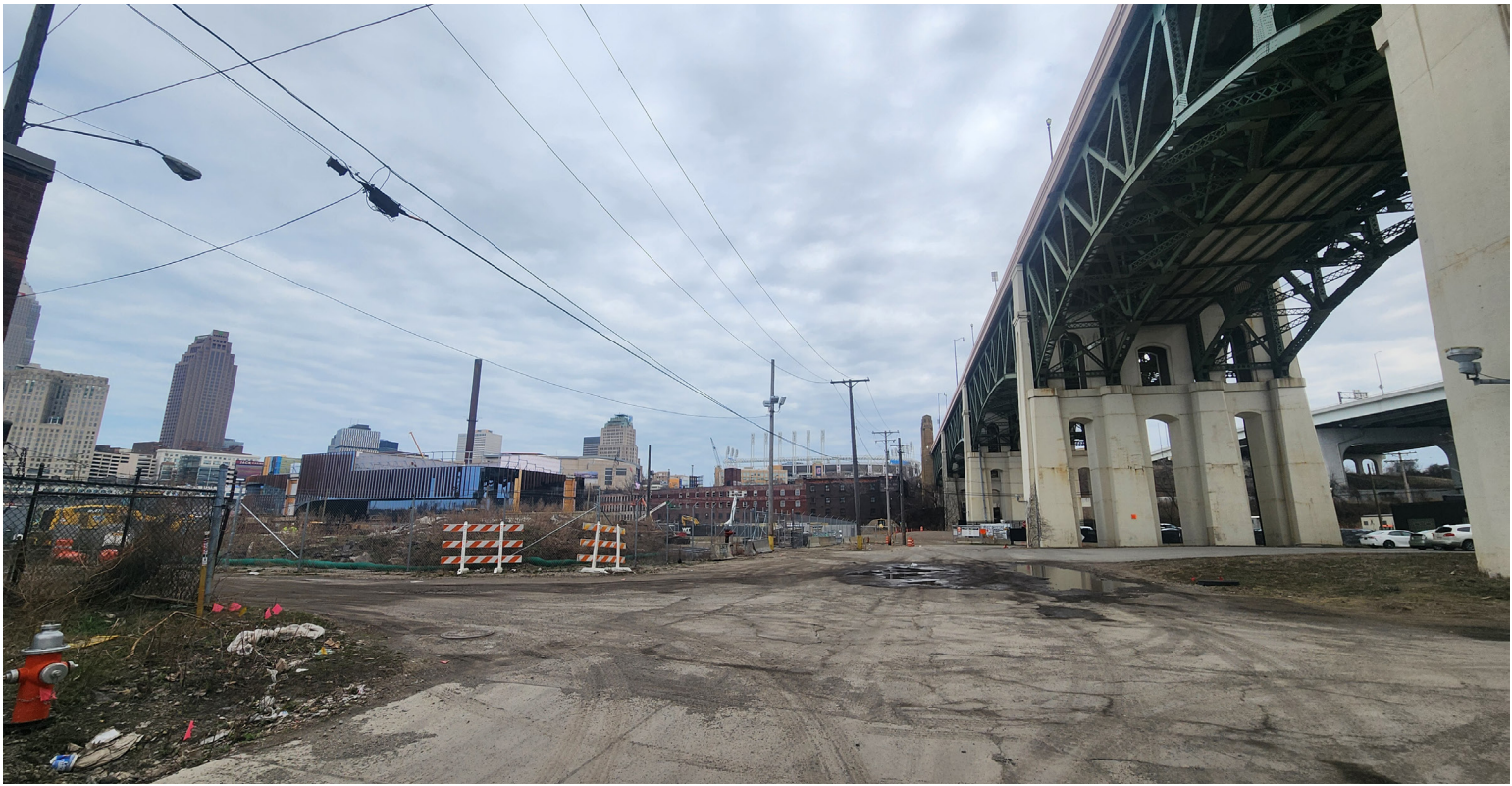
3 CENTRAL AVE VIEW TO THE EAST
