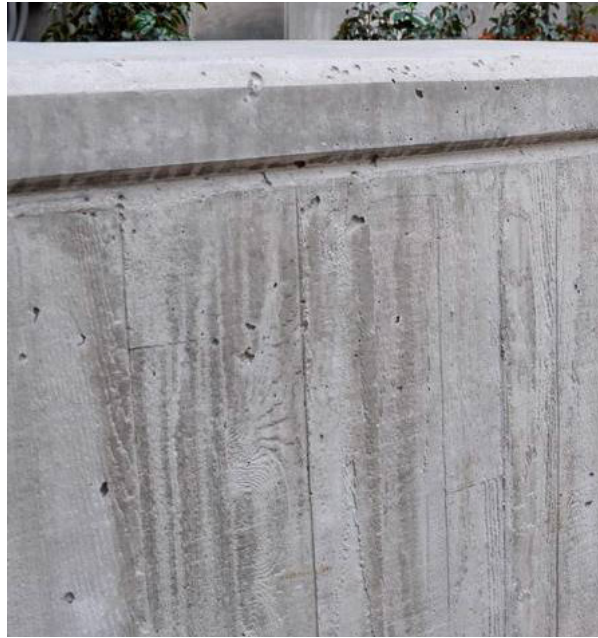
CIP Concrete Seatwall Formliner Finish, Boardform Pattern
