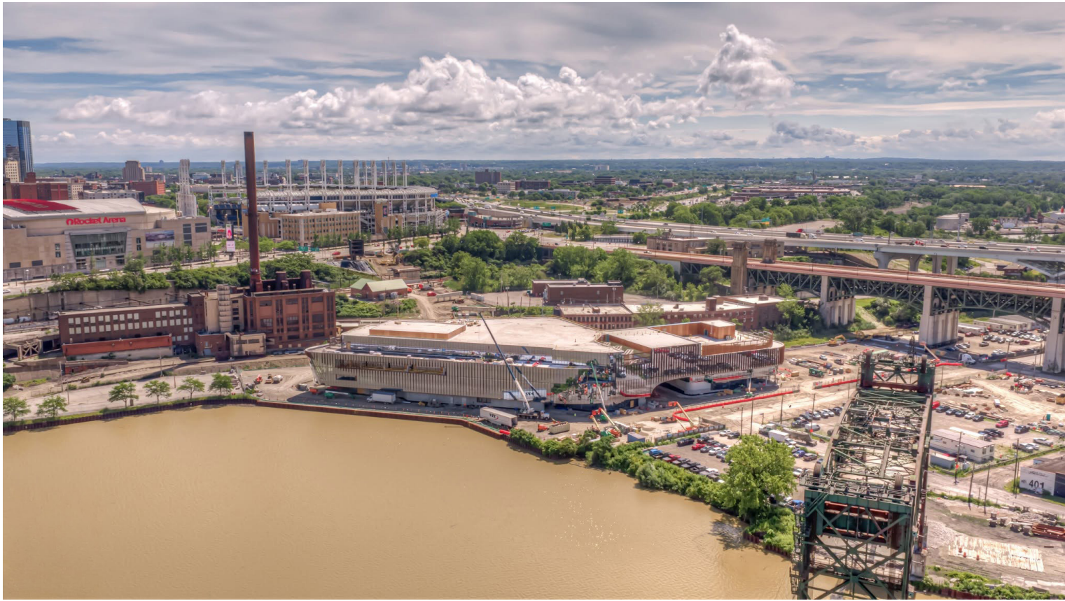
2 AERIAL FROM WEST
