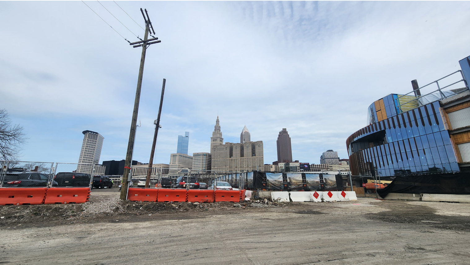
1 FROM NORTHEAST CORNER AT PROPOSED ENTRY PLAZA
