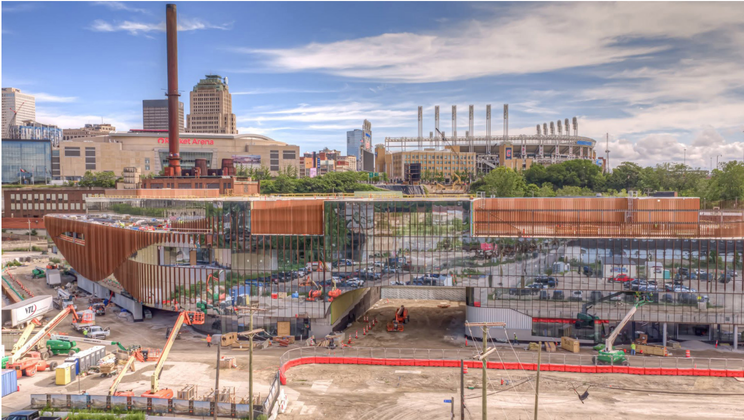
1 AERIAL FROM STONES LEVEE LOOKING EAST TOWARDS EAGLE AVE.
