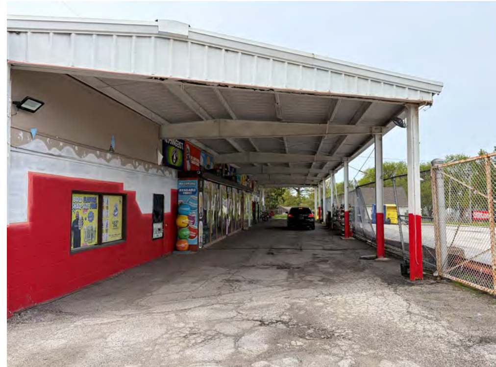
Drive-Thru Site & Other Signage
