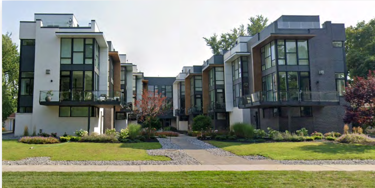
9505 Lake Avenue 10 units, Lake Avenue (0.3 miles)
