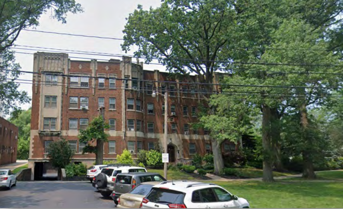
1210 West Blvd (20 units)
