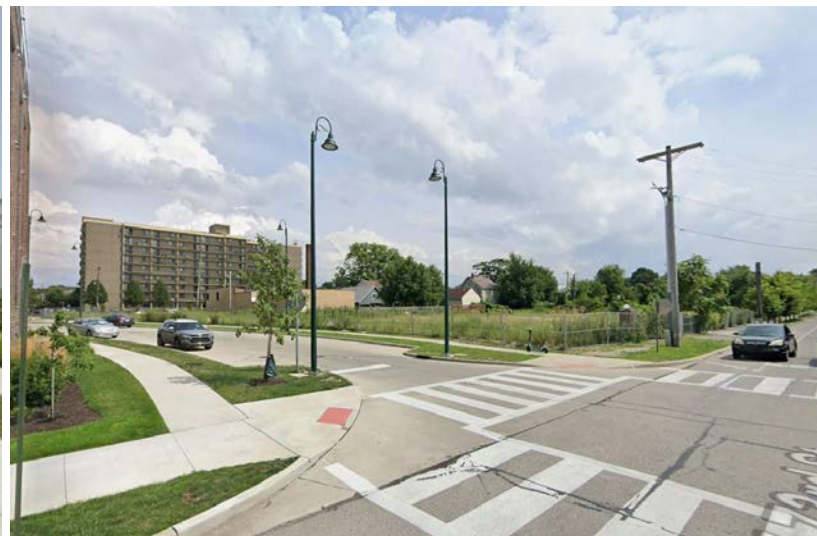
View of Site From Northwest (Corner of Battery Park Blvd & West 73rd Street)
