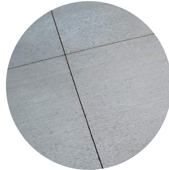
BROOM FINISH CONCRETE Sidewalks
