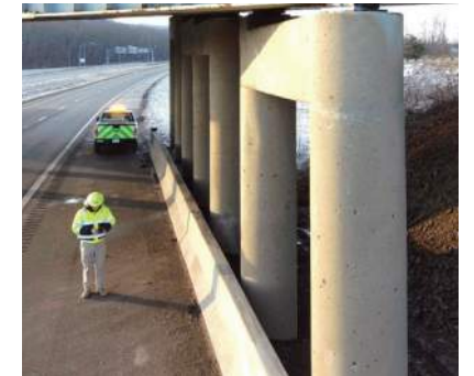
4 Piers | Round column, pier cap, concrete
