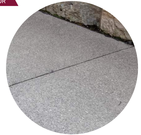
BUFF WASH CONCRETE Sidewalk @ W. 3rd / Eagle Intersection
