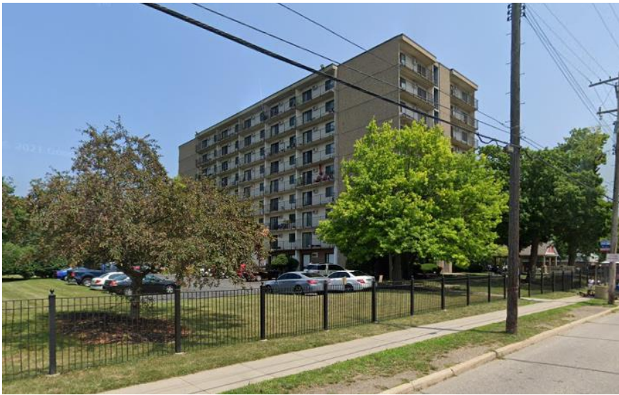
Kingsbury Tower – Apartment building
