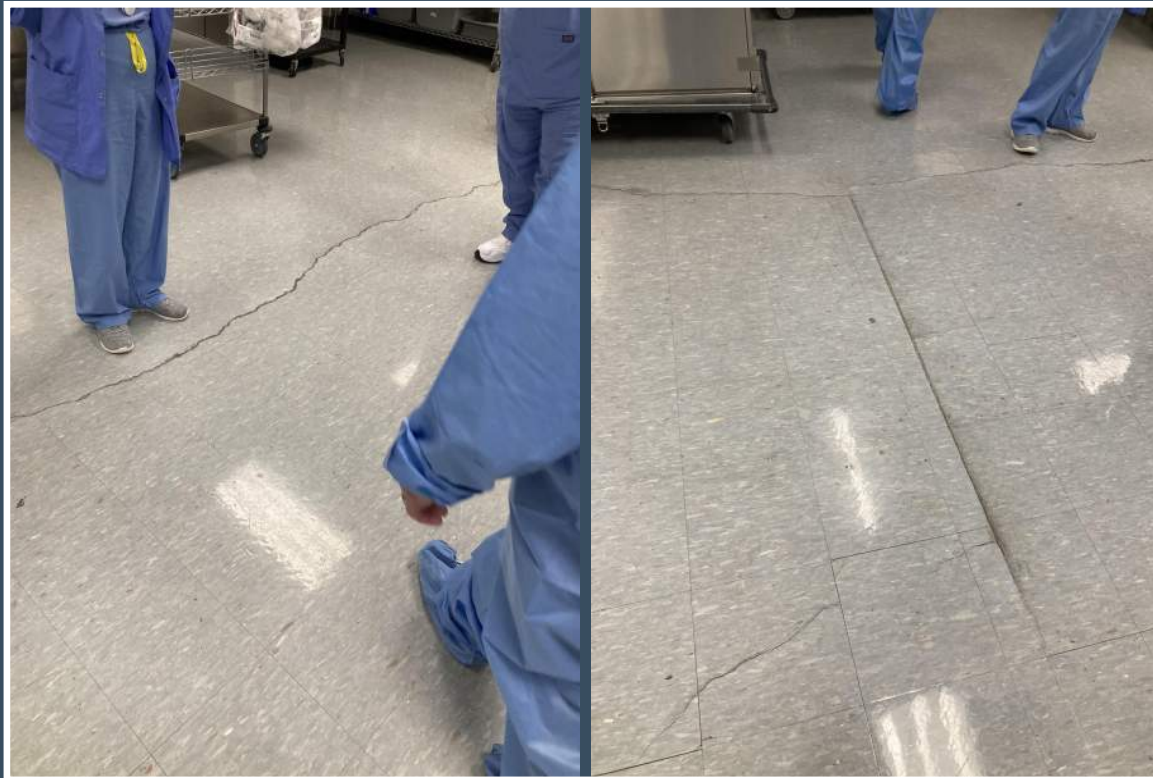
EXISTING BASEMENT FLOOR IMAGES OF THE PYRITIC SHALE PRIOR TO EXCAVATION
