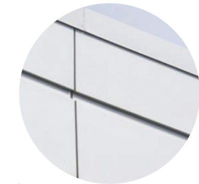
01 PREFINISHED METAL PANEL - METALIC FINISH
