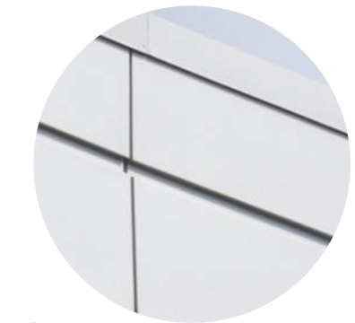
01 PREFINISHED METAL PANEL - METALIC FINISH
