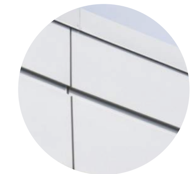
01 PREFINISHED METAL PANEL - METALIC FINISH
