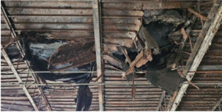
INTERIOR- ROOF STRUCTURE AND DECK CONDITION
