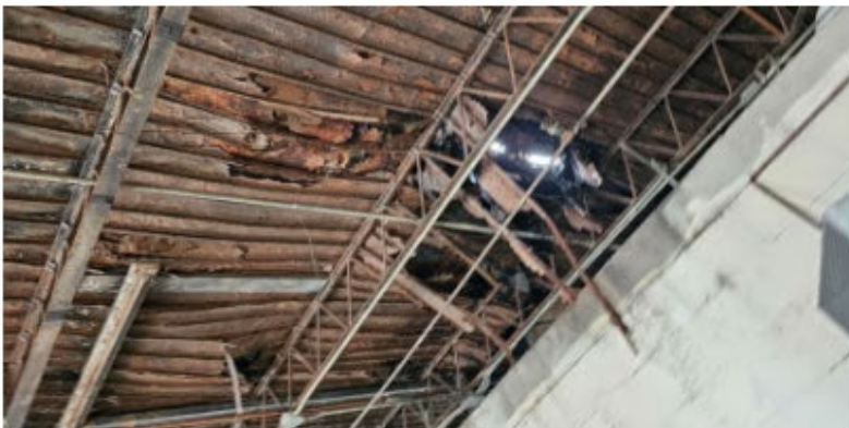
INTERIOR- ROOF STRUCTURE AND DECK CONDITION
