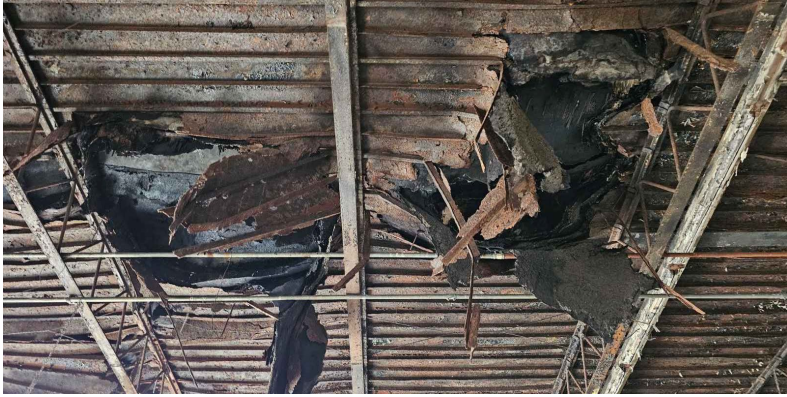
INTERIOR- ROOF STRUCTURE AND DECK CONDITION
