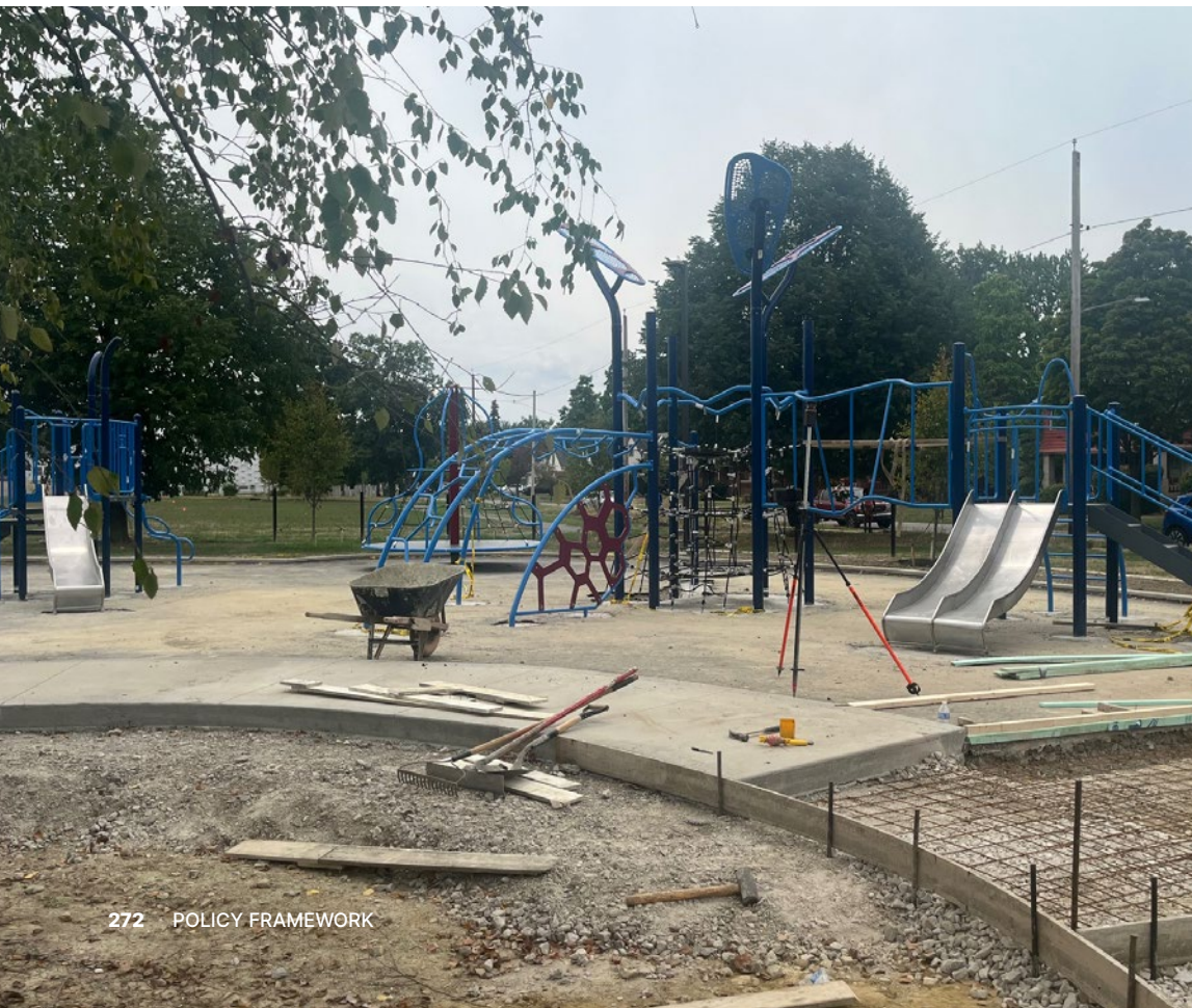
Construction in Glendale Park. Source: City of Cleveland.
