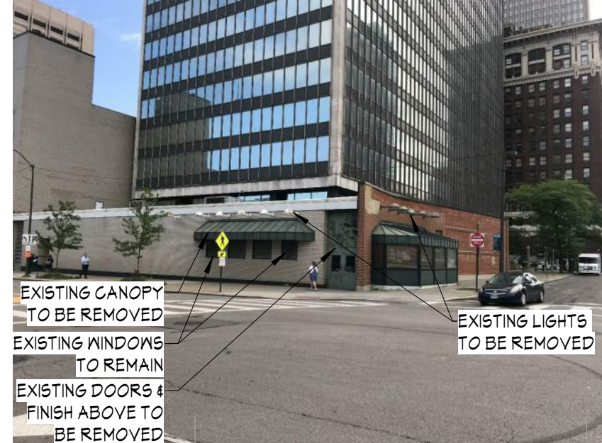
EXTERIOR PHOTOGRAPH #2 - EXISTING CONDITIONS
