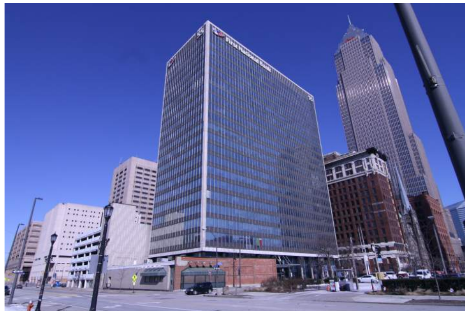
PHOTOGRAPH 01 - CONTEXT VIEW FROM SOUTHWEST
