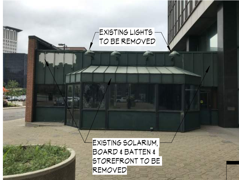
EXTERIOR PHOTOGRAPH #3 - EXISTING CONDITIONS
