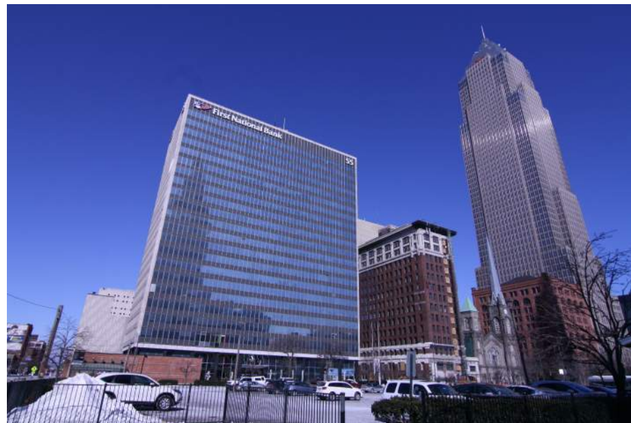
PHOTOGRAPH 02 - CONTEXT VIEW FROM SOUTH
