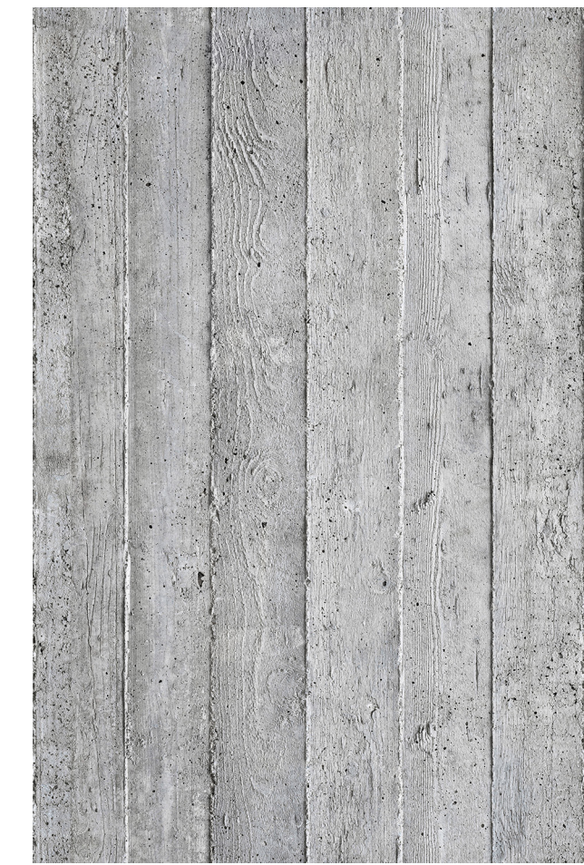
BOARD FORMED CONCRETE CONC-1
