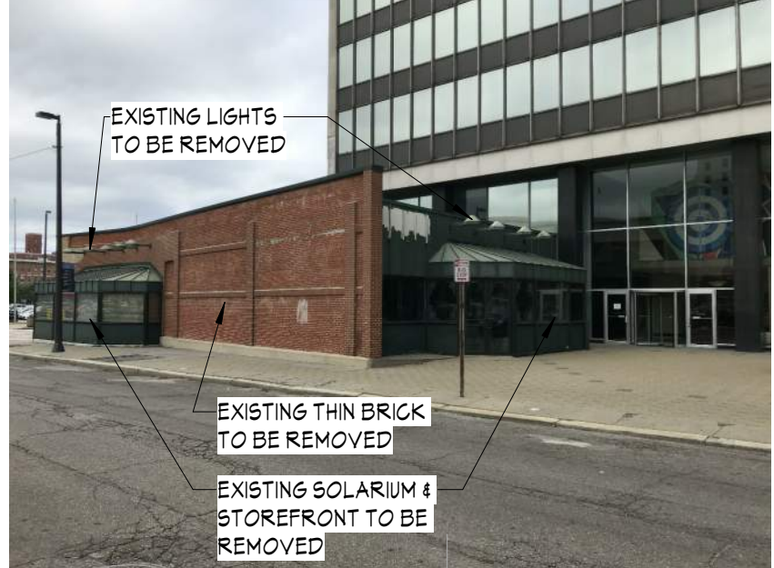
EXTERIOR PHOTOGRAPH #1 - EXISTING CONDITIONS
